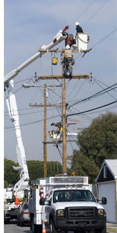
for telephone lines. Telephone lines attach to a steel strand found on the lower part of this spot on the utility pole.
